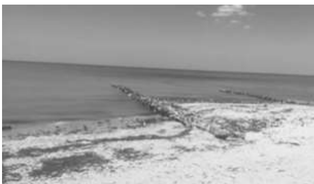
Erosion mitigation, Mexico
