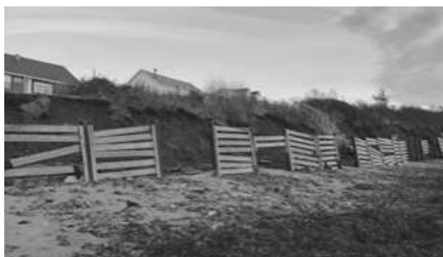
Erosion mitigation, Canada
