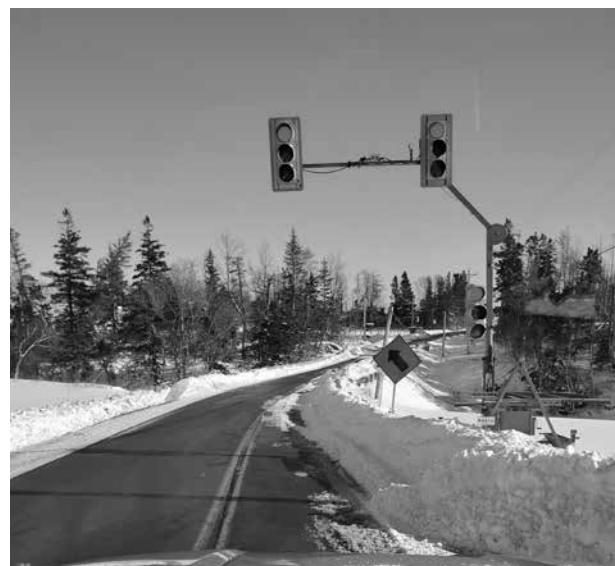
Temporary traffic lights at Murphy Creek, Cape John Road.
